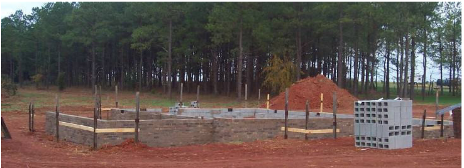
Construction after week 3—the foundation is complete
